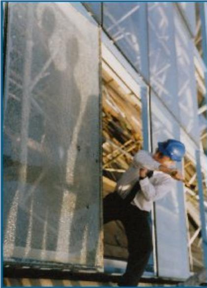
SUPATINT CLEAR SAFETY FILM is designed to hold shattered glass in place when broken.
